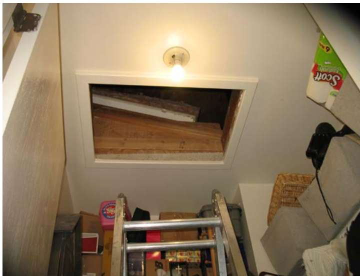
FACTs Photograph of the Attic Access
