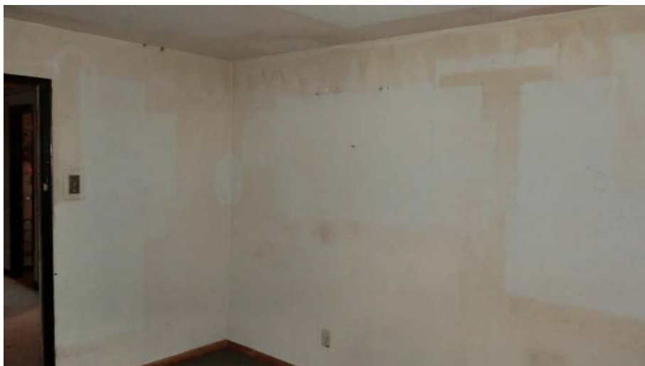
Iodine Staining Basement Northwest Bedroom
