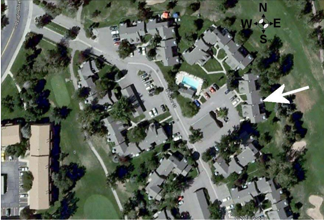
Photograph 1 General Building Layout (Subject property indicated by the white arrow)
