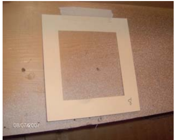
Sample location M-07502.21-08, underneath side of stairs
