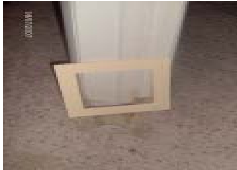
Threshold between first floor northwest bedroom and hall
