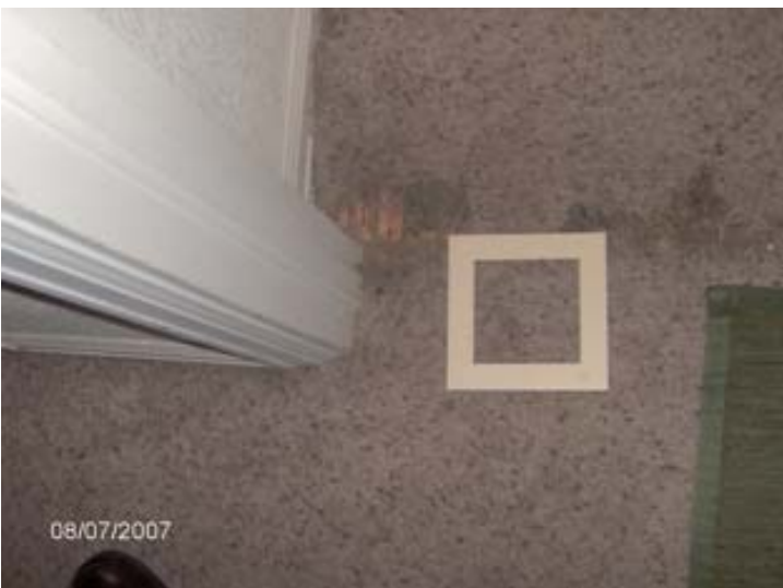
Threshold between basement hall and southeast room
