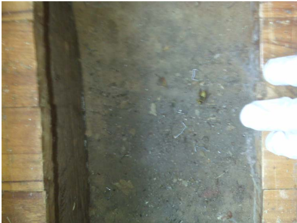
Photograph 2 Duct Interior Northeast Corner of Family Room
