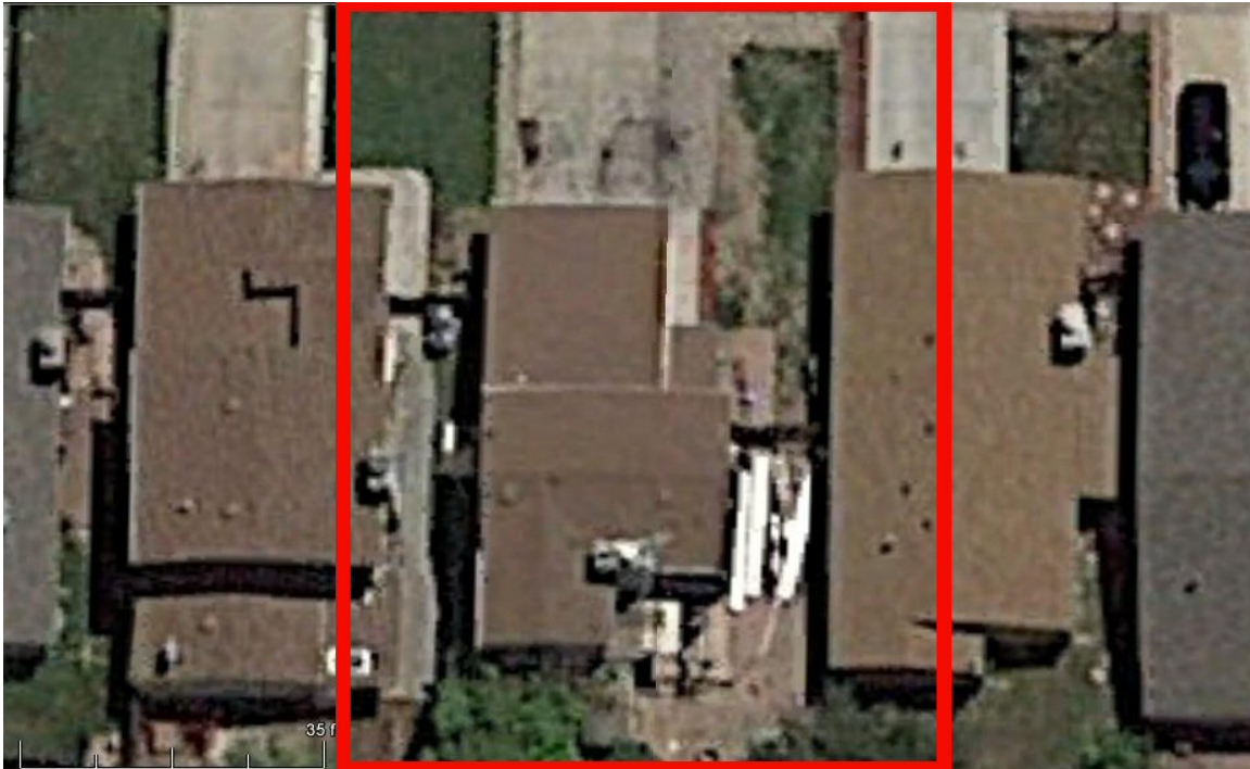
Photograph 7 11767 Grant Street June 2, 2014 15
