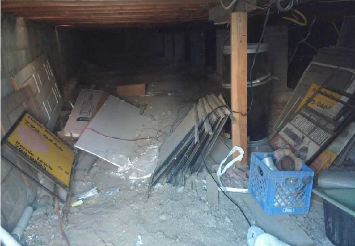
Photograph 3 Photograph of Crawlspace Post Remediation Report
