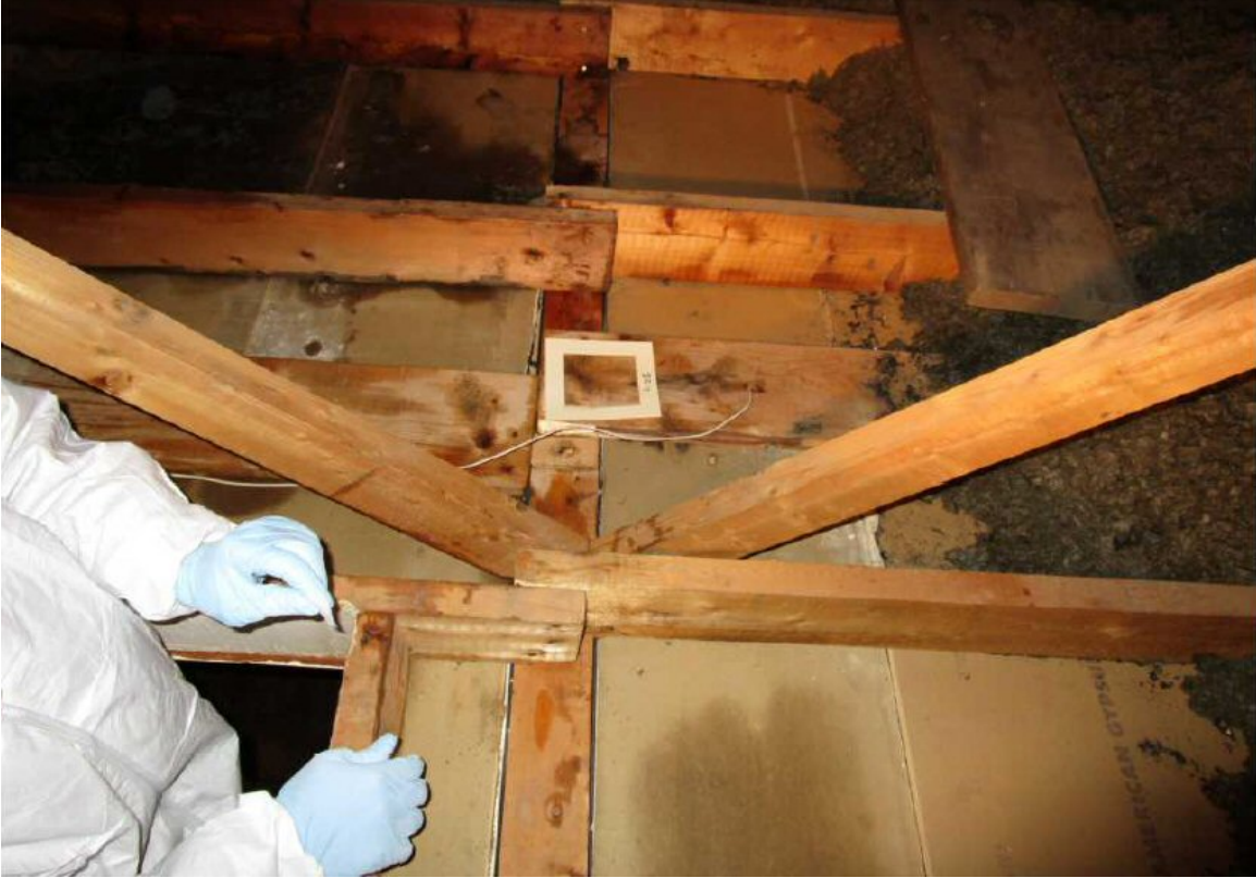
Photograph 4 Photograph of Crawlspace Post Remediation Report
